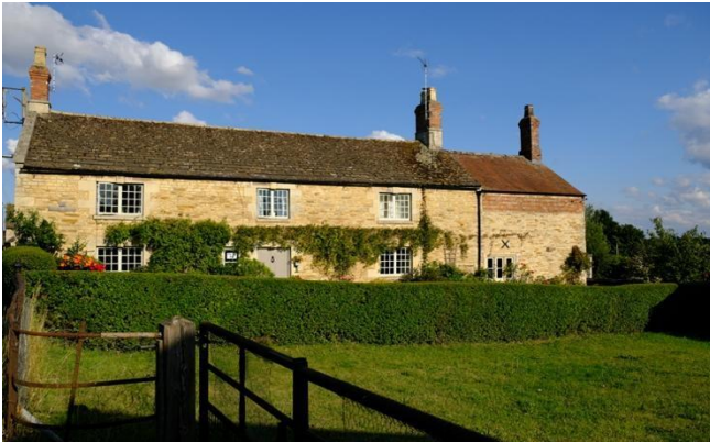
Picture 3 North Luffenham Farm House
